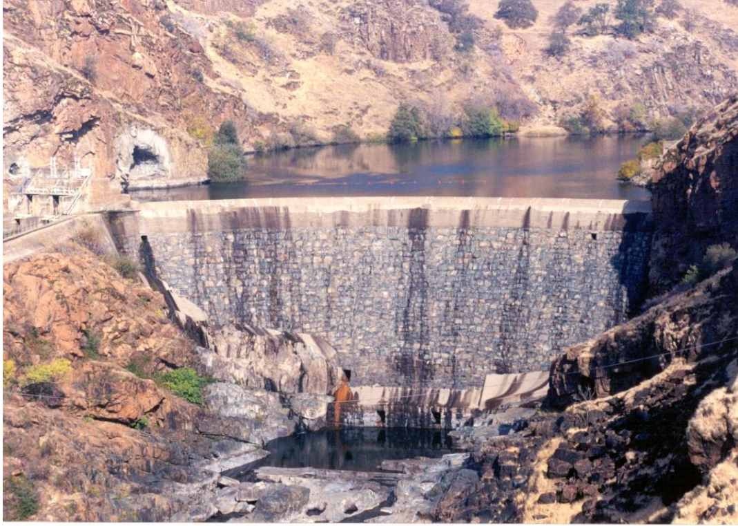
View of La Grange Diversion Dam (built 1893)
