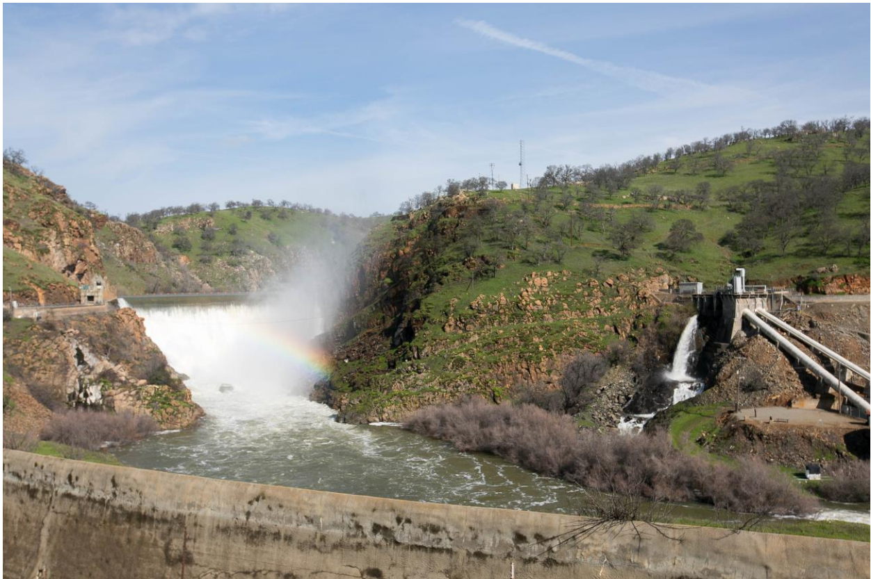
View of La Grange Diversion Dam during overtopping, TID hydrogenation facility shown on the right
