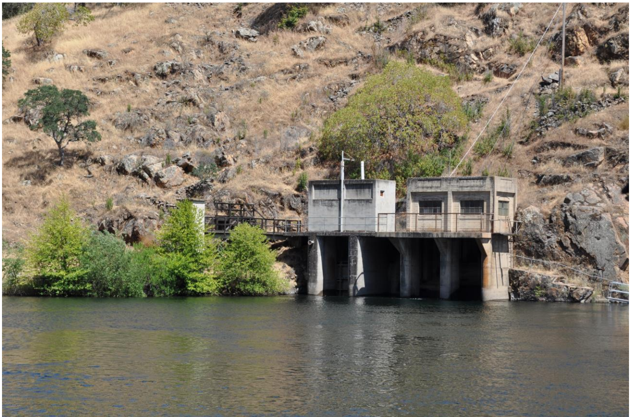
TID Diversion facility to TID Main Canal from La Grange Diversion Dam
