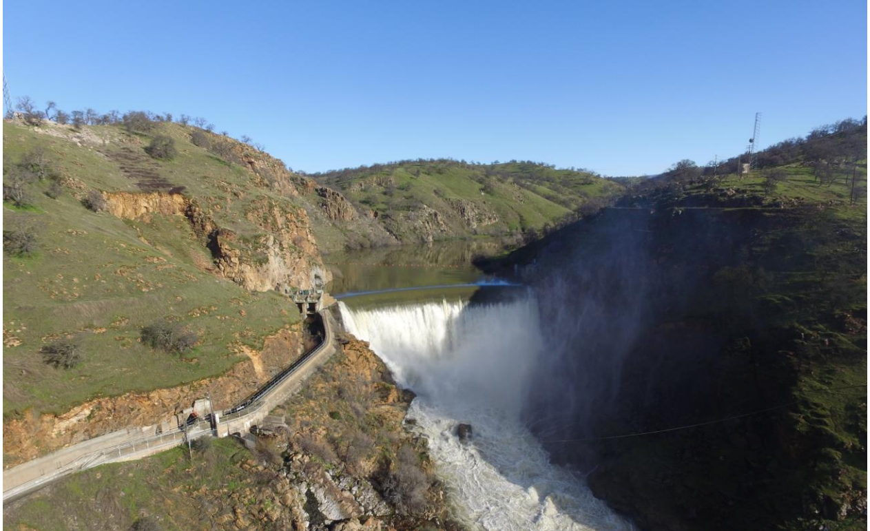
La Grange Diversion Dam, MID diversion facility located on the left side of Diversion Dam
