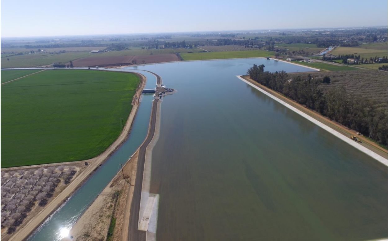
MID Main Canal and Regulating Reservoir
