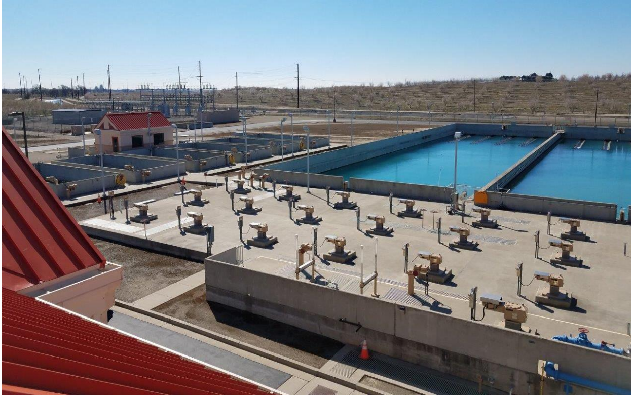
MID Water Treatment Facility
