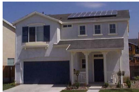
Figure 1 Roof Mounted PV System
