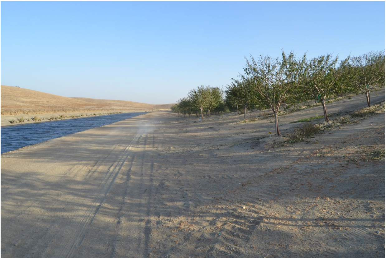
Photo 10. MID Upper Main Canal Potential Ag Runoff Location
