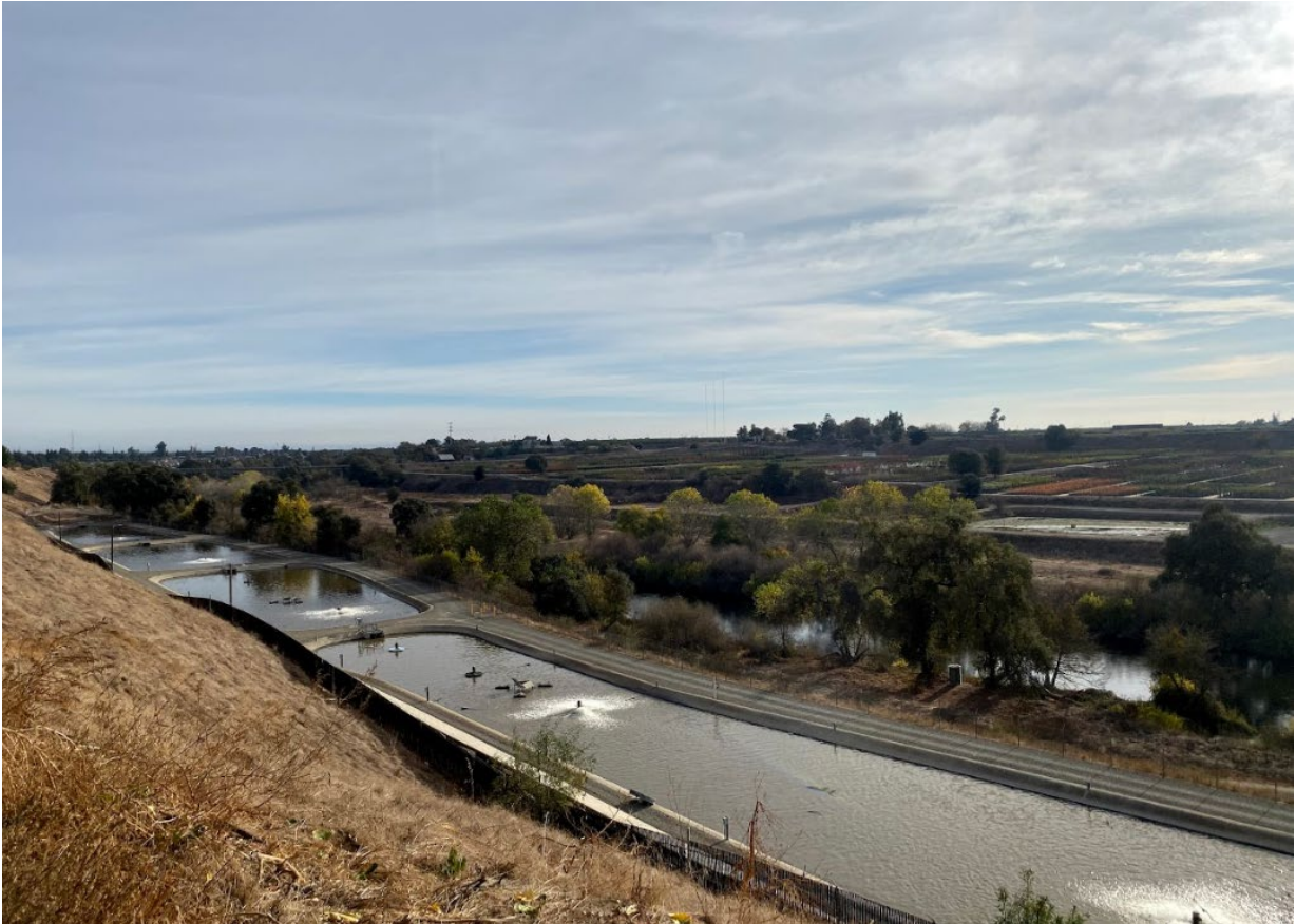
Photo 16. Waste Water Treatment Plant
