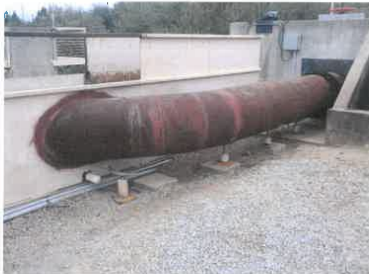
Figure A-1. Adding a 30" pipe to the head of the flume to increase the capacity into the flume (left)
