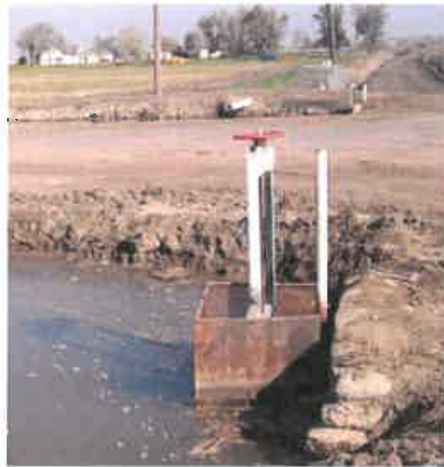
Figure B-11. Correct height of stilling well to match top of gate frame. However, the diameter is too small. Steel pipe material is good
