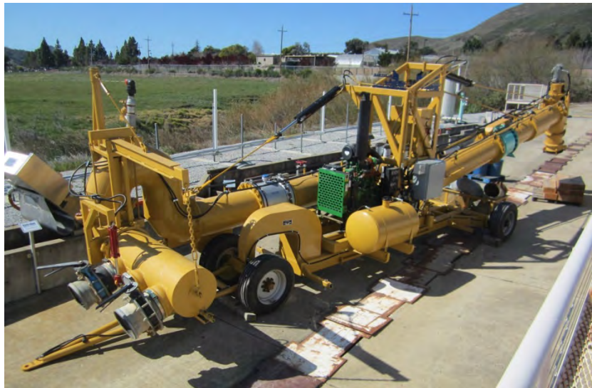
Figure 3. Pumping system for IID jack gate characterization
