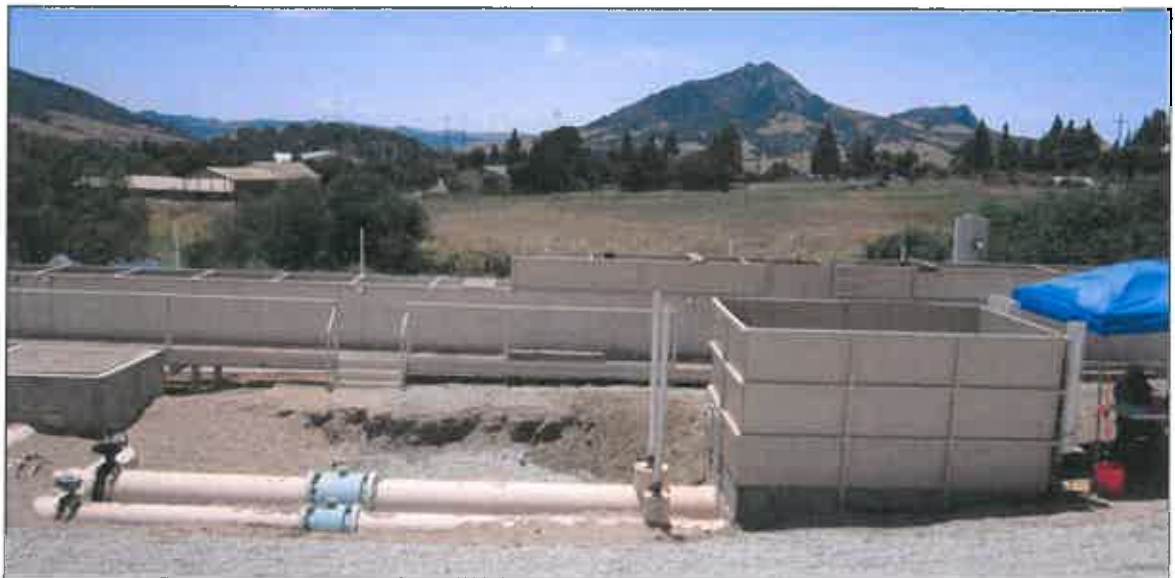
Figure A-6. Completed testing setup after construction.
