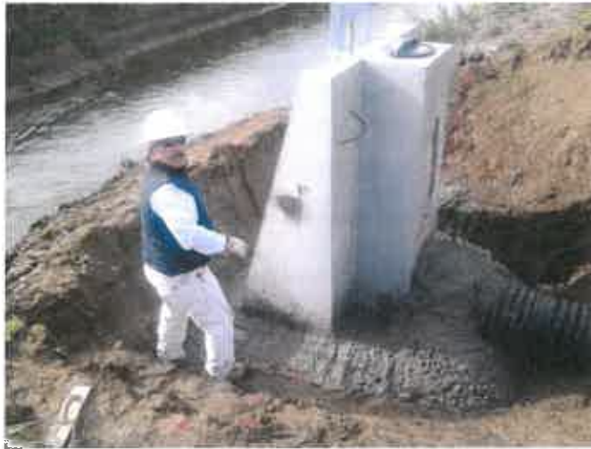
Figure B-15. Installation of GCID meter gate
