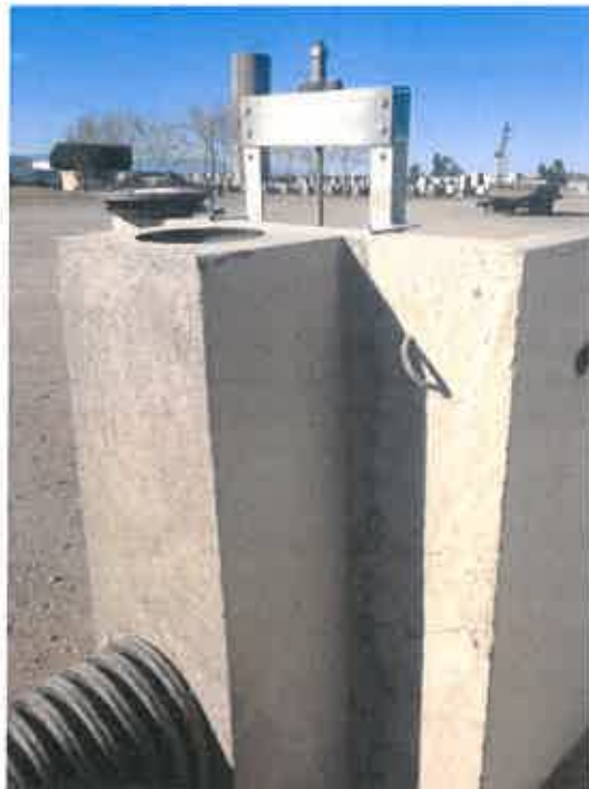
Figure B-13. GCID meter gate at Briggs
