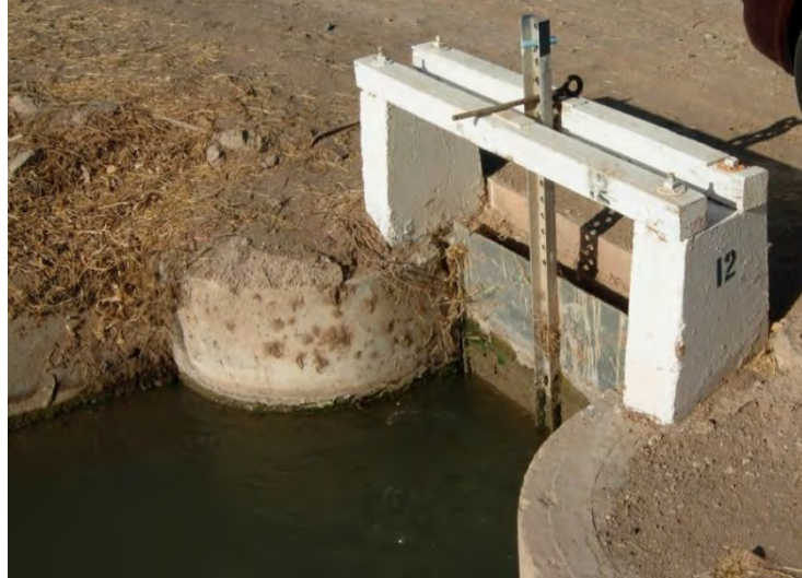
Figure 2. A typical IID jack gate
