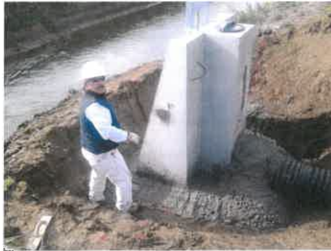
Figure B-15. Installation of GCID meter gate
