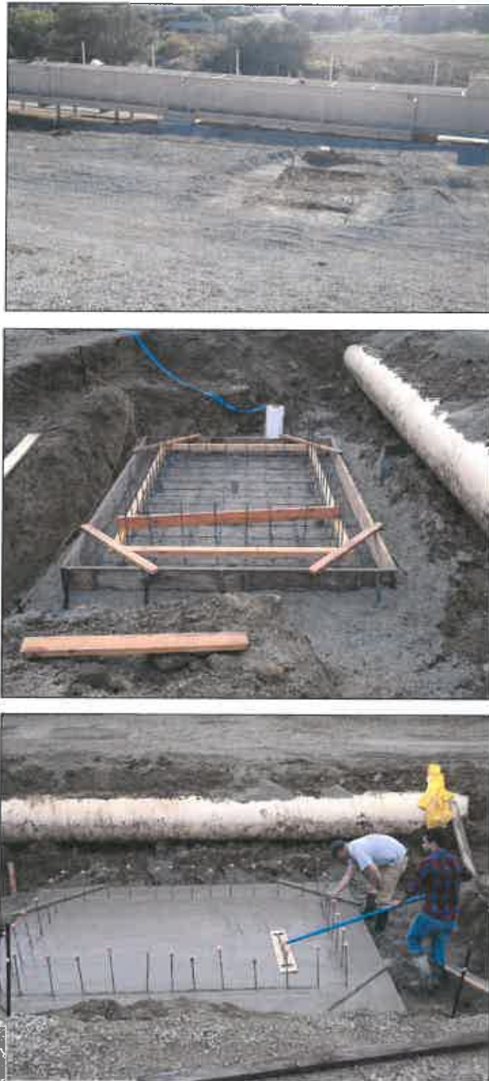
Figure A-3. Initial construction of main spill box that the meter gate pipeline drains into.
