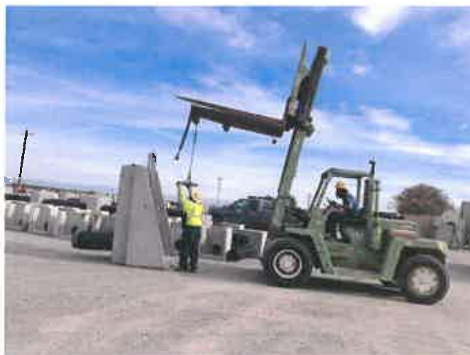
Figure B-14. Pre-cast metergate ready for transport
