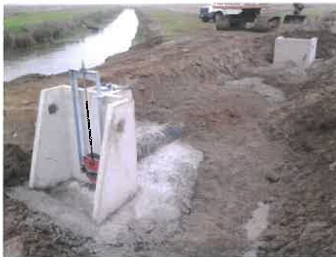
Figure B-16. Final concrete for GCID meter gate, showing downstream pre-cast outlet box.
