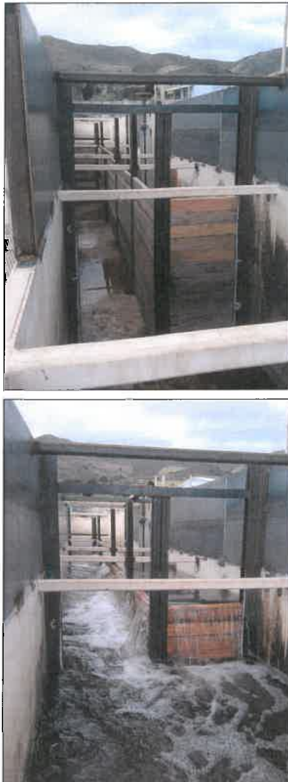
Figure A-5. Weir in flume to maintain the water level upstream of the gate. The photos show a longer weir than was actually used. Only the two bays on the downstream end were used in the actual testing.
