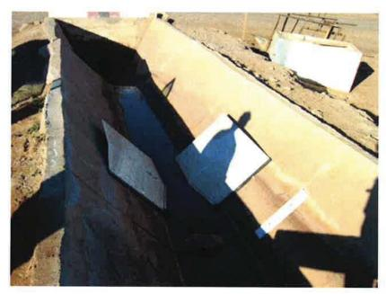
Figure 3. Side contractions rather than a traditional "Replogle Flume". Designed by USBR, Yuma. The rocks are not part of the design.
